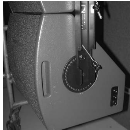
(6) Installation du second I12XT.
